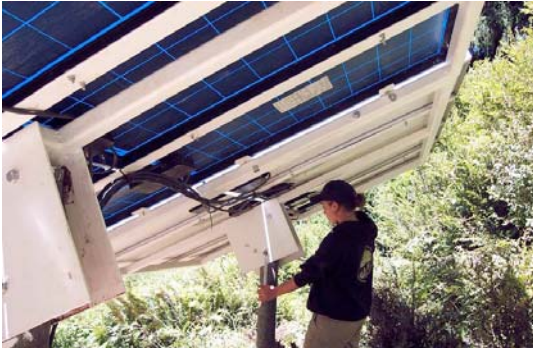
HSU UNPEPP intern adjusts PV rack for summer setting at Espa Lagoon.
