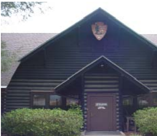
Chattahoochee Headquarters building, one of five assessed buildings
